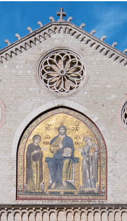
Cathedral, detail of the façade
